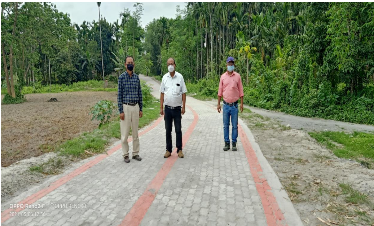
Construction of approach road at Koilamoila Bazar to Kalamati under Assam Darshan in Chirang District for the year 2019-20(Completed)
