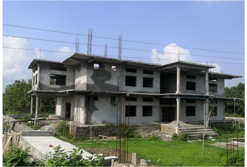
Under construction Office of the Kajalgaon Municipal Board, Kajalgaon
