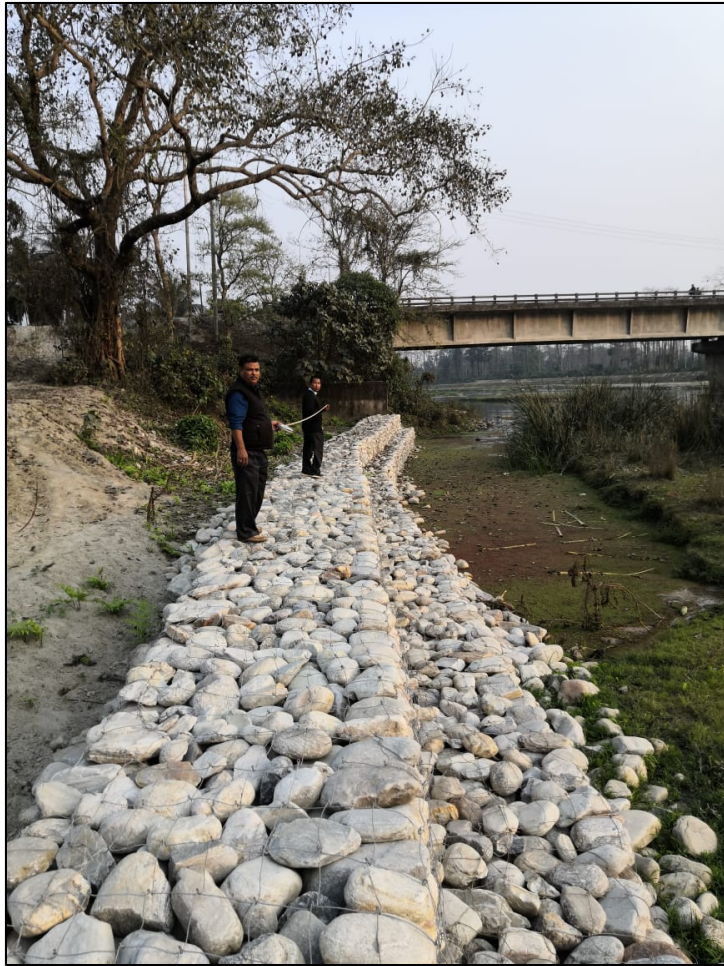
Inspection of work at Bijni MB
